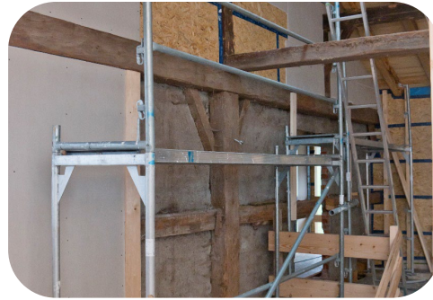
Remodeling/ renovations only
