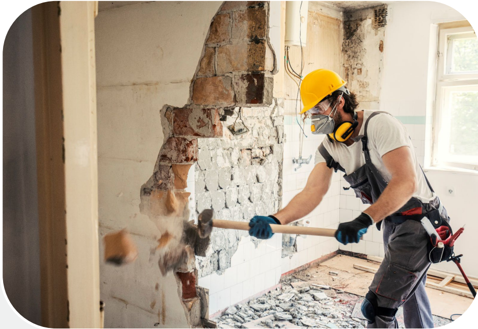
Ongoing construction activity
